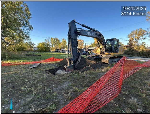
Photo 7: View of soil excavation sampling location
