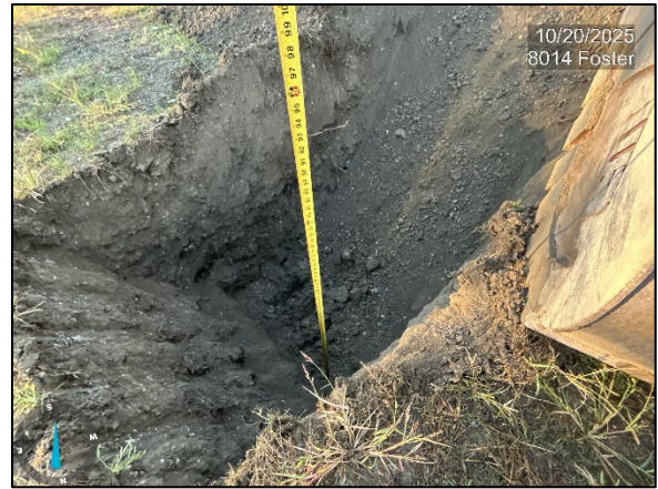
Photo 8: View of excavation pit where soil sample was collected
