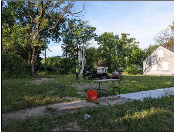
Photo 1: Viewing 6760 Brimson during initial soil boring activities
