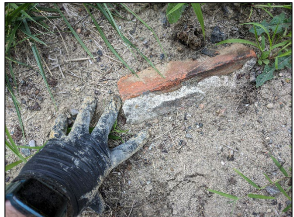
Photo 4: Viewing Building Debris Found at the Surface of the Site.
