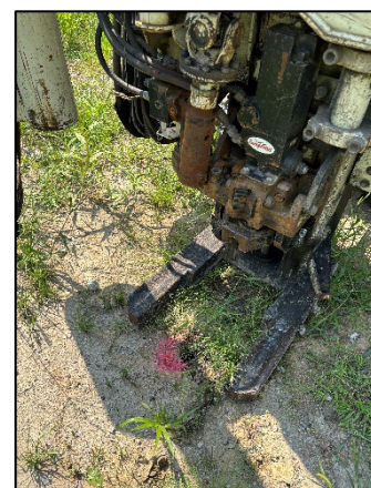
Photo 6: Viewing 3915 SB03 Drilling, Facing West.
