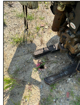
Photo 4: Viewing 3915 SB02 Drilling, Facing West.
