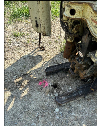
Photo 2: Viewing 3915 SB01 Drilling, Facing West.
