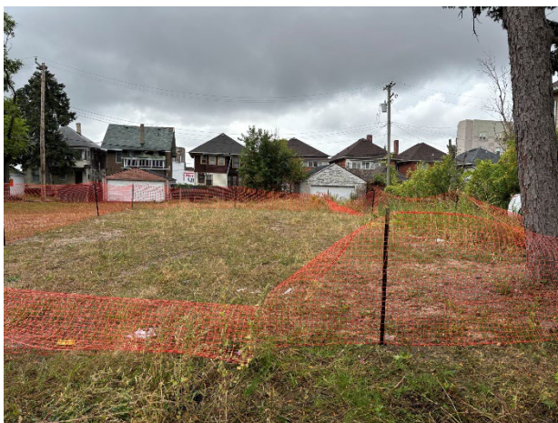
Photo 5. View of Site following TCLP sampling activities
