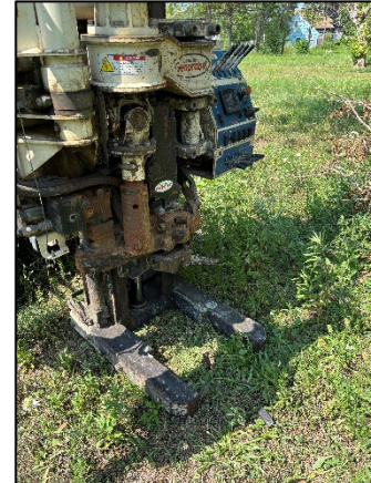
Photo 2: Viewing 14433 SB01 Drilling, Facing West.
