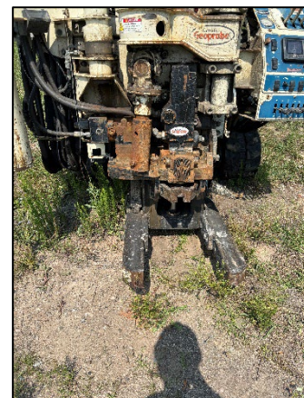
Photo 6: Viewing 14433 SB03 Drilling, Facing West.
