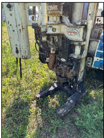
Photo 5: Viewing 14411 SB03 Drilling, Facing East.
