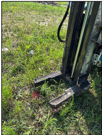
Photo 3: Viewing 14411 SB02 Drilling, Facing East.
