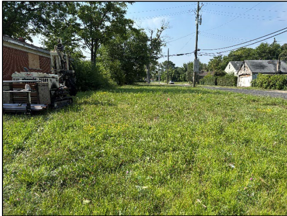
Photo 1: Viewing Site Pre-Drilling at the time of initial soil boring activities
