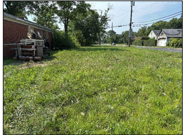
Photo 8: Viewing Site Post-Drilling at the time of initial soil boring activities
