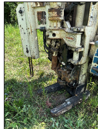
Photo 4: Viewing 14131 SB02 drilling, facing east.
