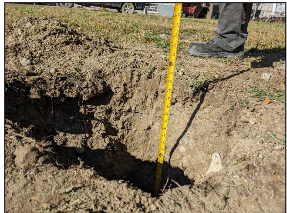
Photo 12: View of the hand augured supplemental soil sample boring location
