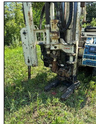
Photo 6: Viewing 14124 SB03 Drilling, Facing Southwest.
