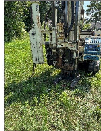
Photo 4: Viewing 14124 SB02 Drilling, Facing Southwest.
