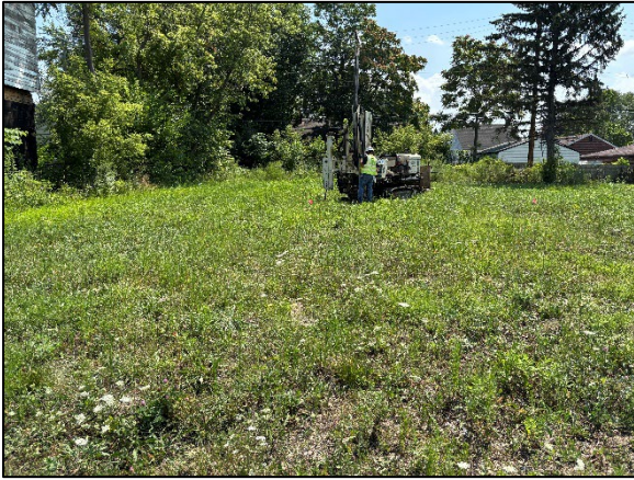
Photo 1: Viewing Site Pre-Drilling, Facing South.
