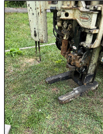
Photo 2: Viewing 14119 SB01 Drilling, Facing West.
