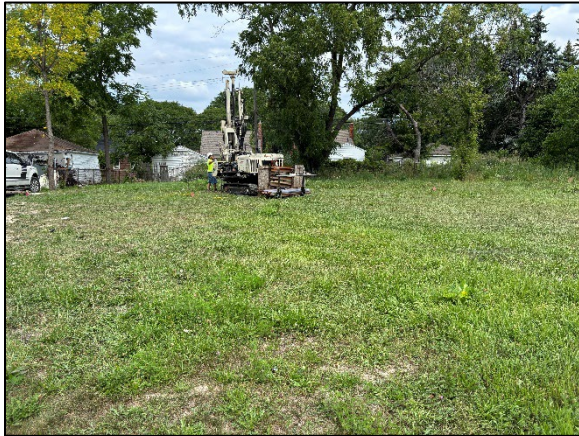
Photo 1: Viewing Site Pre-Drilling at the time of initial soil boring activities, Facing North.
