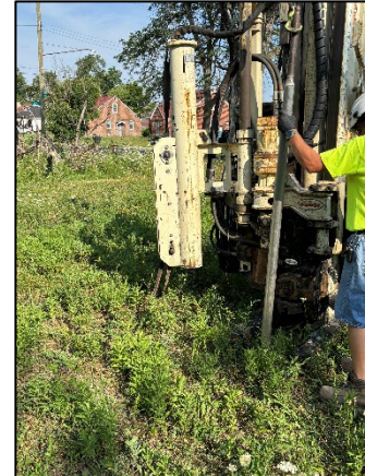
Photo 2: Viewing 14118 SB01 Drilling, Facing Northwest.
