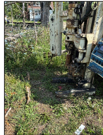
Photo 4: Viewing 14118 SB02 Drilling, Facing Northwest.
