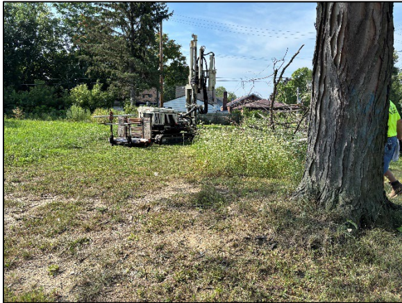
Photo 1: Viewing Site Pre-Drilling, Facing South.
