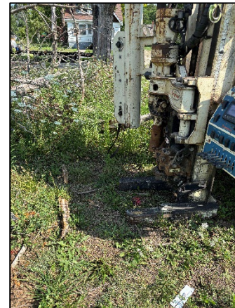
Photo 4: Viewing 14110 SB02 Drilling, Facing North.
