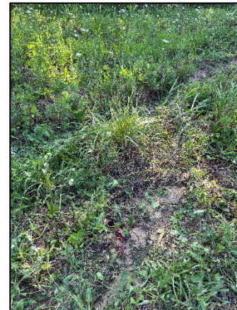
Photo 4: Viewing 14005 SB02 Drilling, Facing West.
