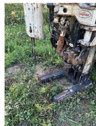
Photo 6: Viewing 14005 SB03 Drilling, Facing West.
