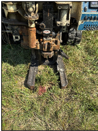
Photo 7: Viewing 13800 SB03 Drilling, Facing West.
