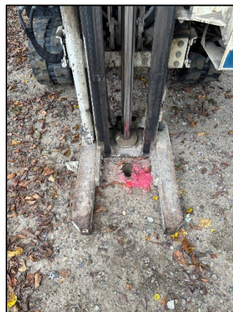
Photo 2: Viewing 13726 SB01 Drilling, Facing East.
