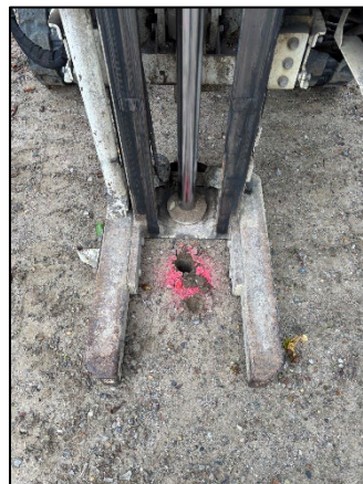
Photo 4: Viewing 13726 SB02 Drilling, Facing East.
