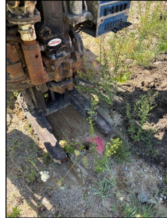
Photo 2: Viewing 13568 SB01 Drilling, Facing Northeast.
