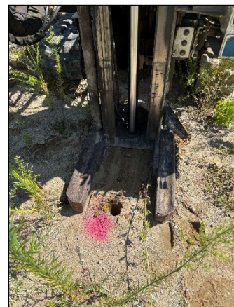
Photo 6: Viewing 13568 SB03 Drilling, Facing Northeast.
