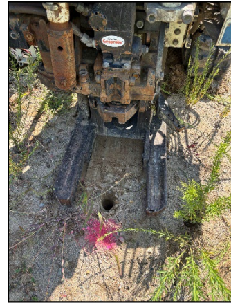
Photo 4: Viewing 13568 SB02 Drilling, Facing Northeast.
