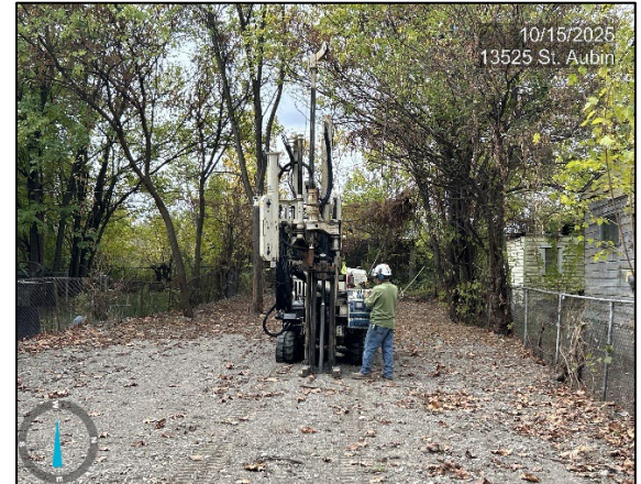
Photo 4: Viewing advancement of 13525 St. Aubin SB-3
