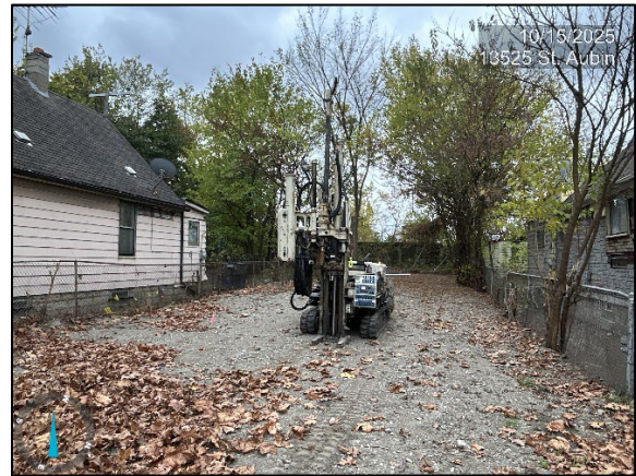
Photo 2: Viewing advancement of 13525 St. Aubin SB-1
