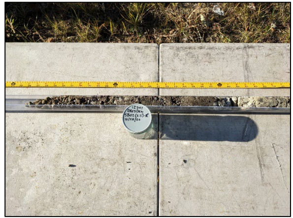
Photo 8: View of soil recovery at the time of supplemental soil sampling activities
