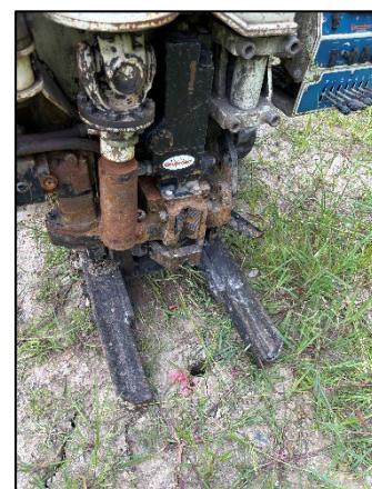
Photo 6: Viewing 12053 SB03 Drilling, Facing East.
