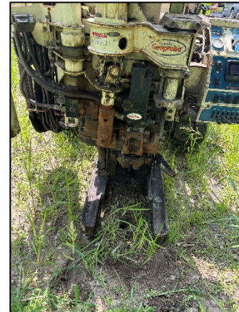
Photo 2: Viewing 12053 SB01 Drilling, Facing East.
