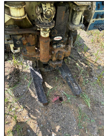
Photo 4: Viewing 12027 SB02 Drilling, Facing East.
