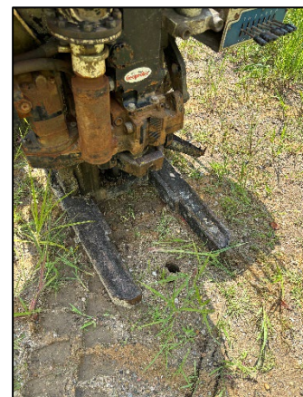
Photo 6: Viewing 12027 SB03 Drilling, Facing East.
