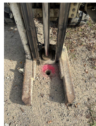
Photo 6: Viewing 11944 SB03 Drilling, Facing Northeast.
