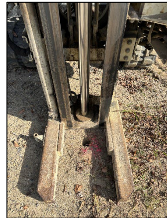
Photo 4: Viewing 11944 SB02 Drilling, Facing Northeast.
