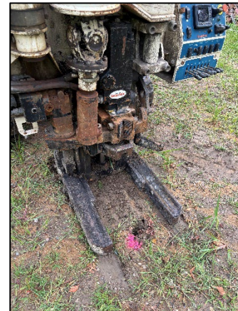
Photo 4: Viewing 11850 SB02 Drilling, Facing West.
