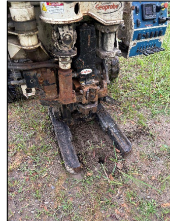
Photo 2: Viewing 11850 SB01 Drilling, Facing West.
