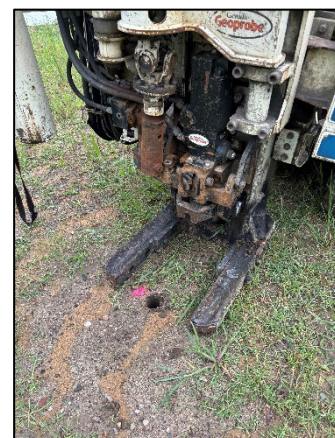
Photo 6: Viewing 11850 SB03 Drilling, Facing West.
