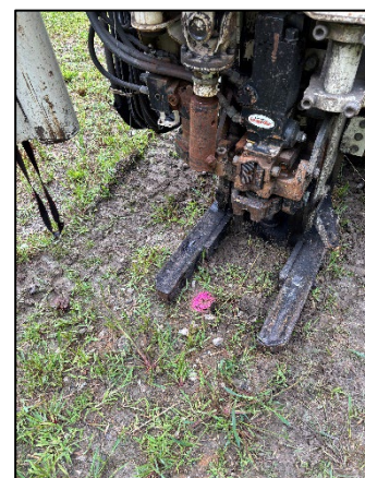
Photo 6: Viewing 11748 SB03 Drilling, Facing East.
