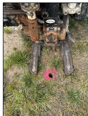
Photo 6: Viewing 11050 SB03 Drilling, Facing Southeast.
