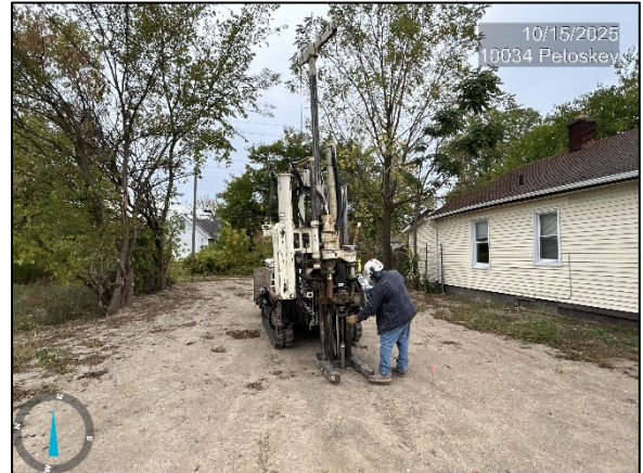
Photo 2: Viewing advancement of 10034 Petoskey SB-1
