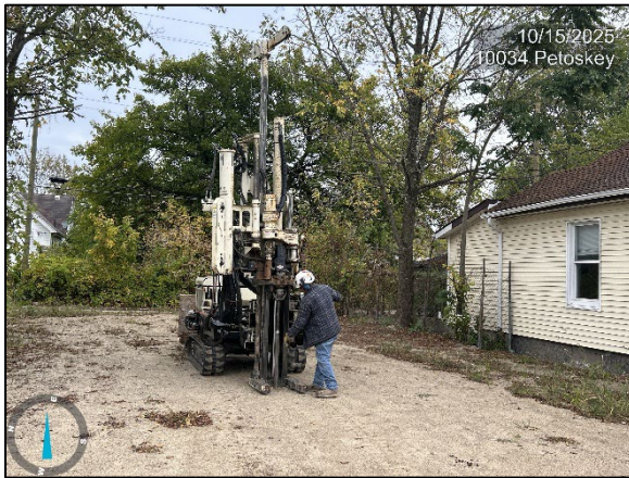
Photo 3: Viewing advancement of 10034 Petoskey SB-2
