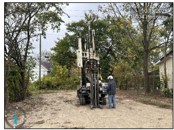
Photo 4: Viewing advancement of 10034 Petoskey SB-3
