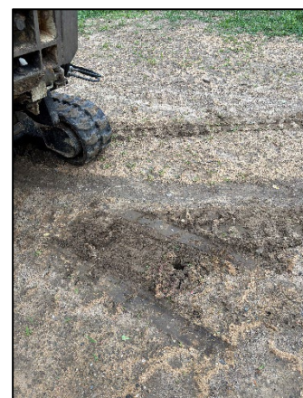
Photo 6: Viewing 12770 SB03 Drilling, Facing Northwest.
