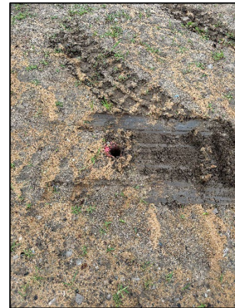
Photo 4: Viewing 12770 SB02 Drilling, Facing Northwest.
