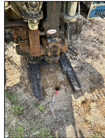
Photo 4: Viewing 11118 SB02 Drilling, Facing East.
