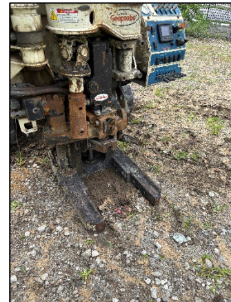
Photo 4: Viewing 12311 SB02 Drilling, Facing Northeast.
