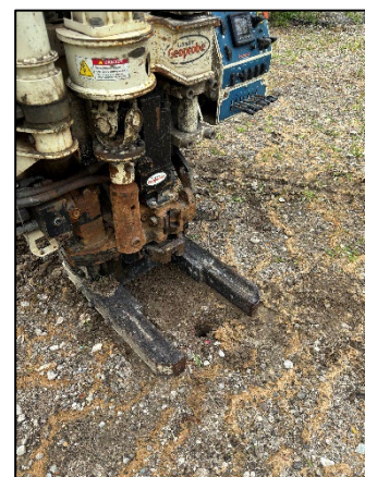
Photo 6: Viewing 12311 SB03 Drilling, Facing Northeast.
