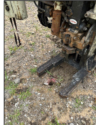
Photo 2: Viewing 12311 SB01 Drilling, Facing Northeast.
