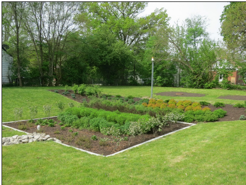
Figure 6: Evergreen Vacant Lot Bioretention
