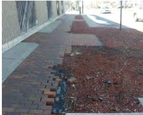
G Failed paving and bare planting beds on Livernois south of 7 Mile.
