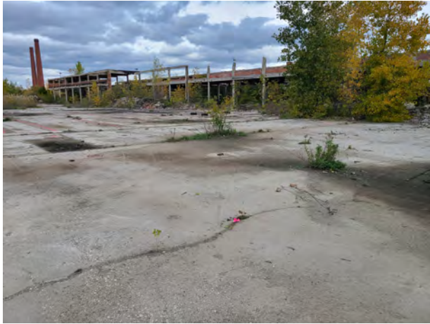
Facing northeast, viewing overall site. Photo taken by Patrick Howe on 10/22/21.
