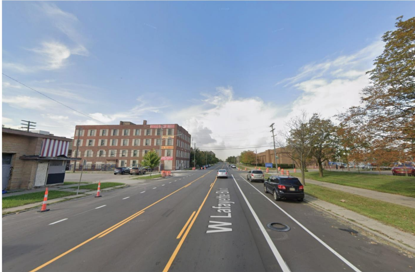
Lafayette, street view at Lafayette Blvd, looking west toward 10th St.
