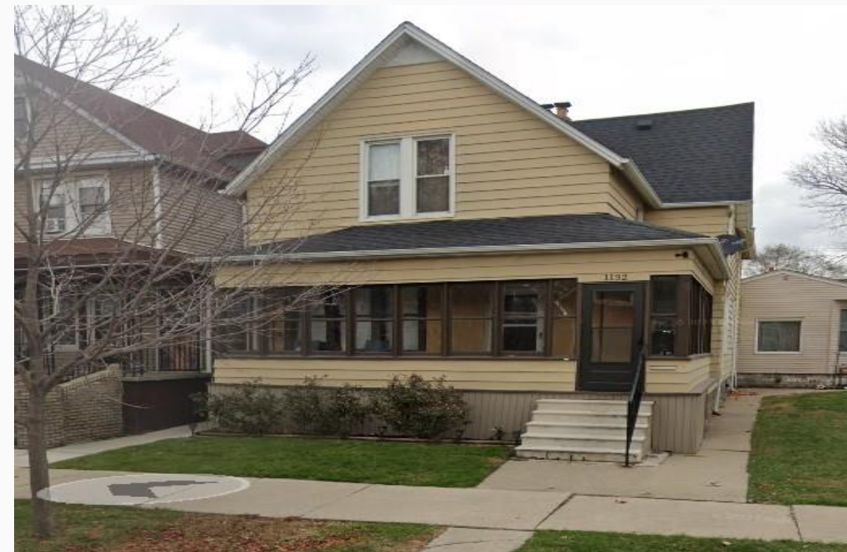
Central Southwest, 4-Unit, Built 1910
