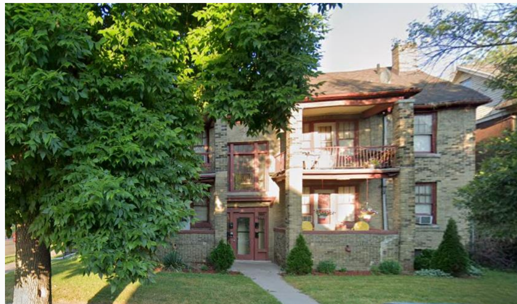
Central Southwest, 12 units
