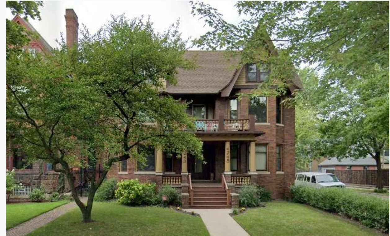
Woodbridge, 4-unit, Built 1909
