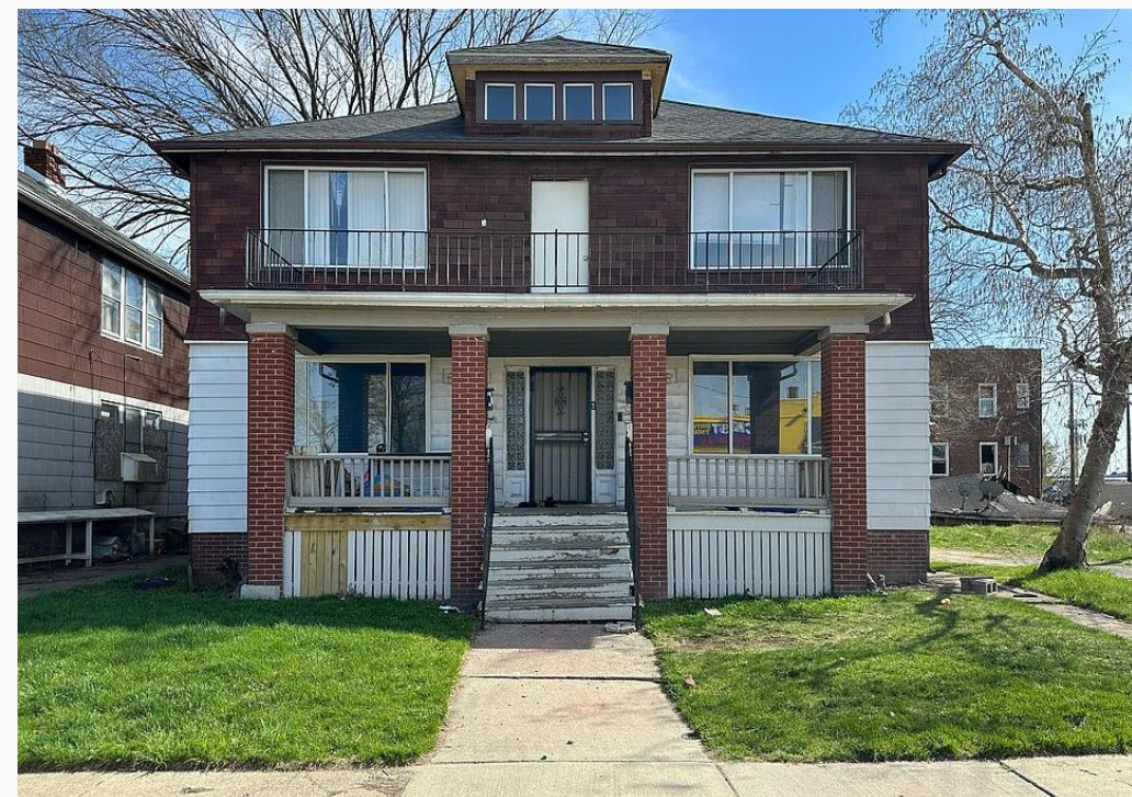
Maple Ridge, 4-Unit, Built 1924
