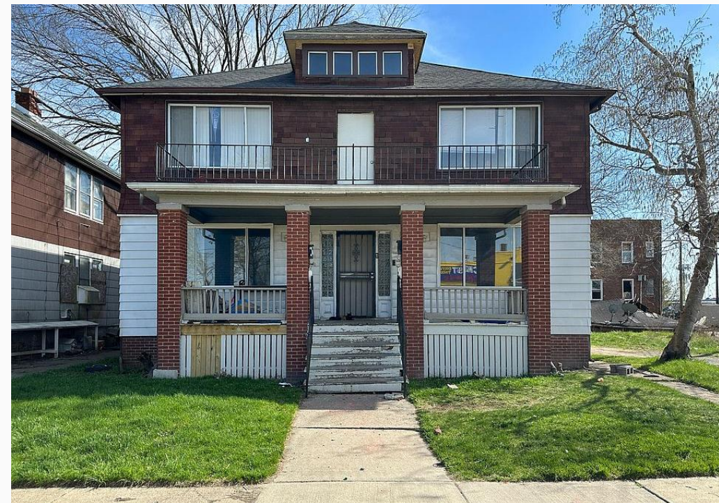
Maple Ridge, 4-Unit, Built 1924
