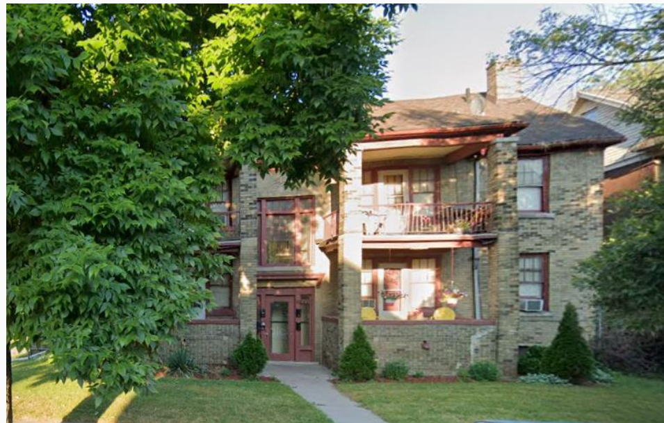
Central Southwest, 12 units
