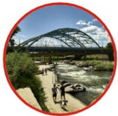
South Platte River Greenway Denver, CO
