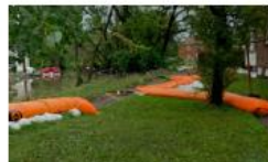
Failed and Relocated Tiger Dams
