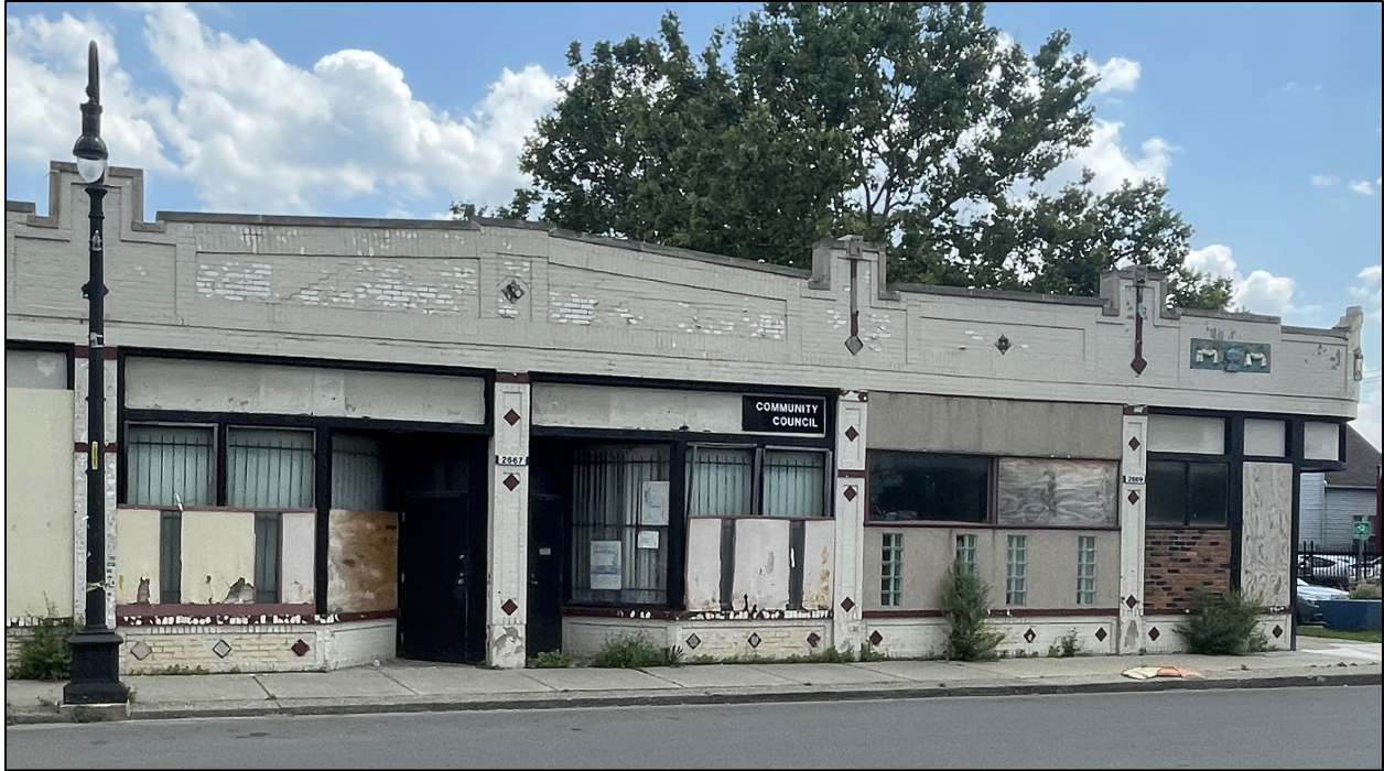
Figure 56. Boarded up windows, peeling paint, brick degradation observed on this vacant, historic commercial building are indications that deferred maintenance is a serious threat. (Kraemer Design Group, 2023)
