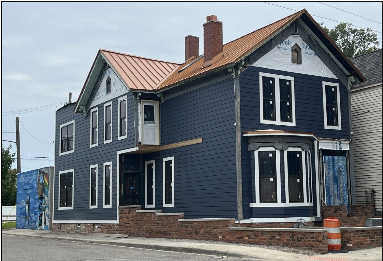
Figure 52. The Lozano House, at 1326 18th Street, was the only residence surveyed. Work is being completed on the house which includes new siding, new windows, and a new roof. (Kraemer Design Group, 2023)
