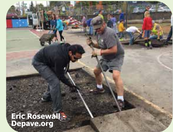
Impervious surface removal
