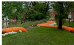
Failed and Relocated Tiger Dams
