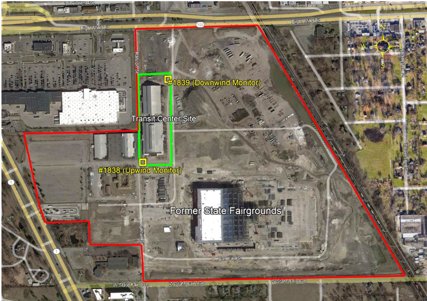
Figure 1 – Monitor Locations at the DDOT Transit Center Construction Site
