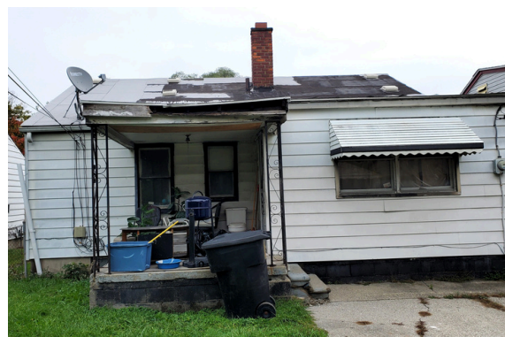
Before Senior Roof Replacement
