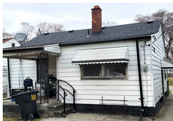
After Senior Roof Replacement
