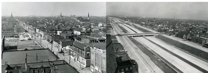
The photograph on the left shows an aerial view of Hastings Street, near Mack Avenue, in 1959. Hastings was once the center of commercial activity for Black Detroit. The photograph on the right, while not the exact vantage point, shows the construction of I-75 just north of the interchange with I-375 in 1961. The Michigan Department of Transportation included these photographs in a presentation on its proposal to remove I-375, built in the 1950s and 1960s for what was then $50 million, and replace it with a boulevard.
