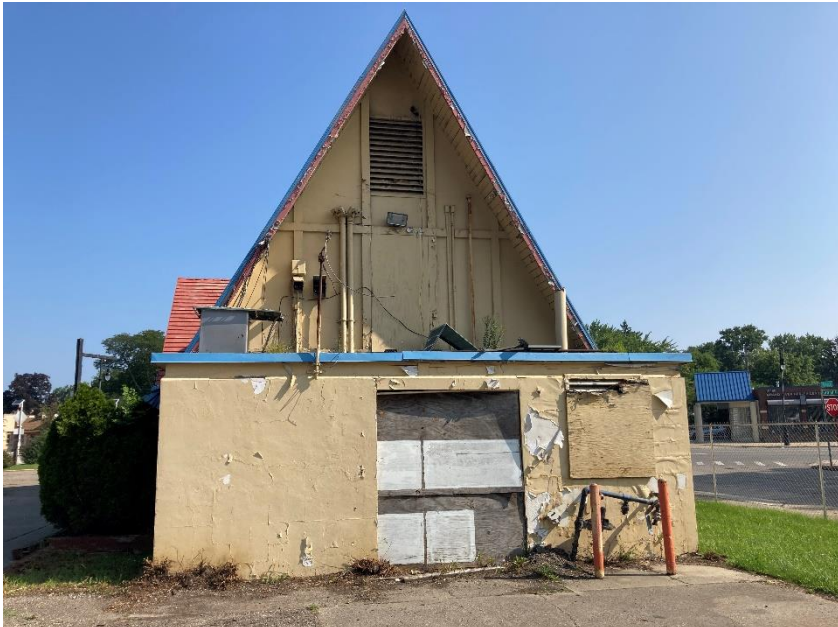
South facing wall of 19505 Grand River Avenue
