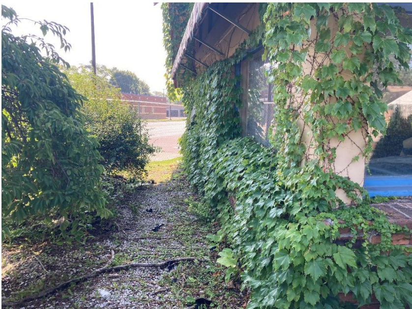
North facing wall of 19505 Grand River Avenue
