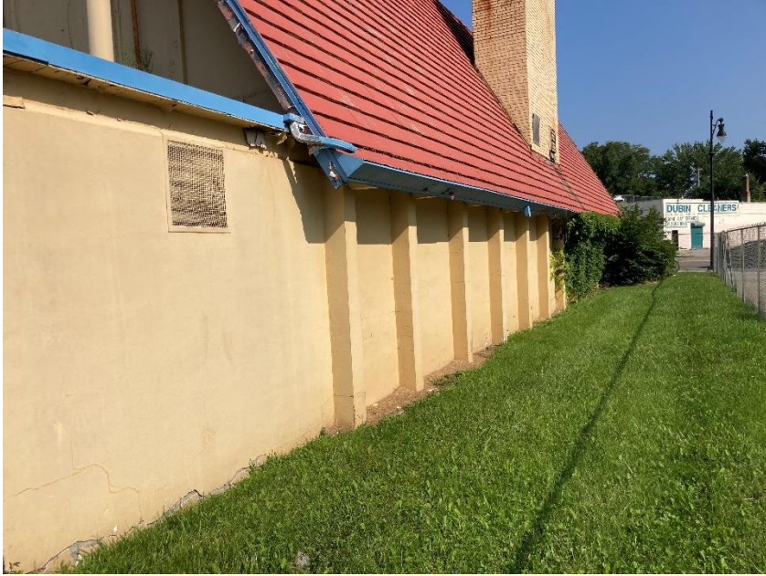
East facing wall of 19505 Grand River Avenue
