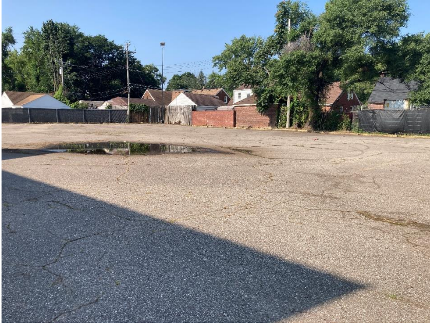
Pavement south and west of the restaurant building
