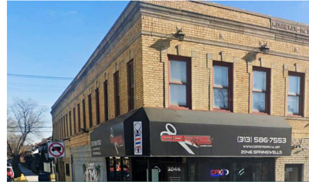
2nd Story Apartment Renovations
