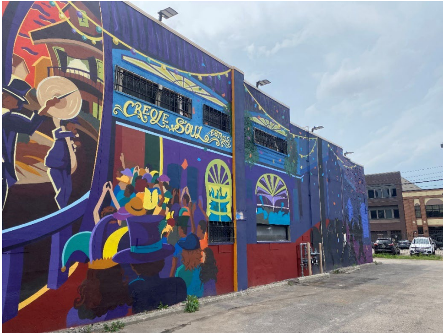
Mural painted on the east façade of the building but not included in the permit application
