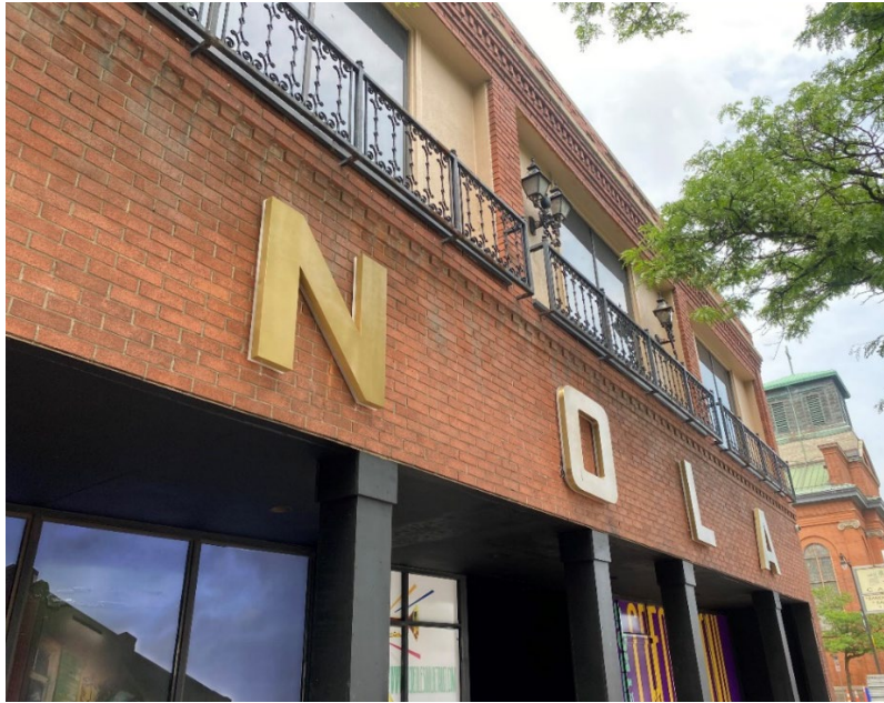
Signage installed on the front (Jefferson) façade of the building without benefit of a permit
